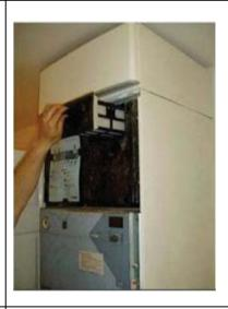
Turn off the NIBE Lift the panel off and pull out the filter.
