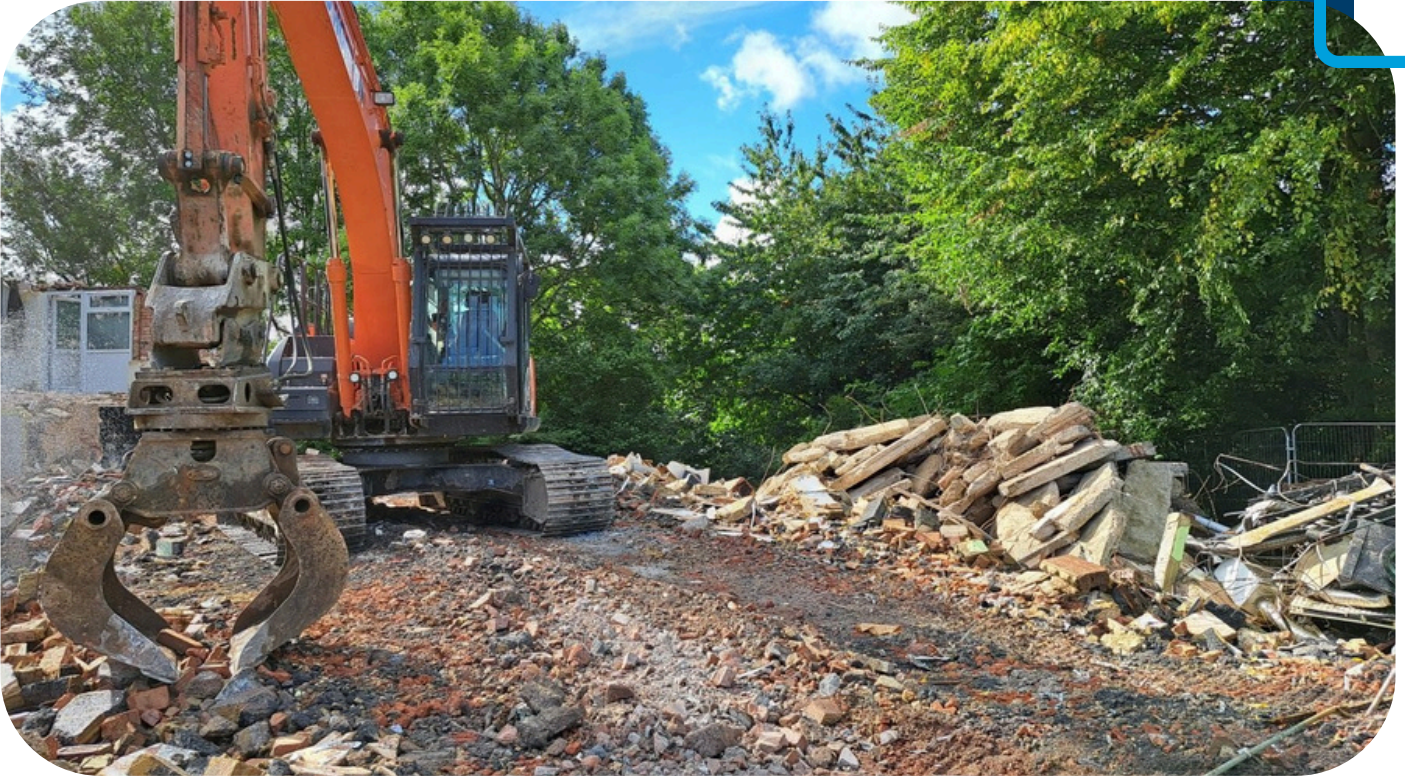
Derelict flats in Warminster being demolished, creating space for 18 new affordable homes.
